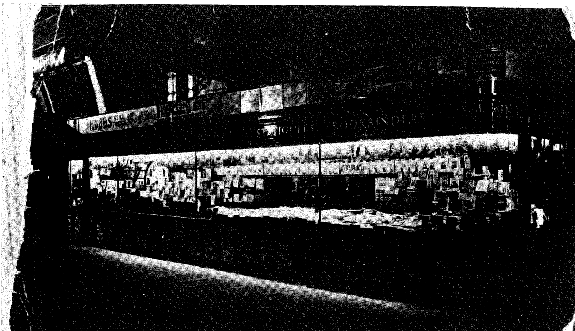
ELECTRICAL INSTALLATION IN BOOKSTALL, ST. PANCRAS STATION (L.M.S.)
