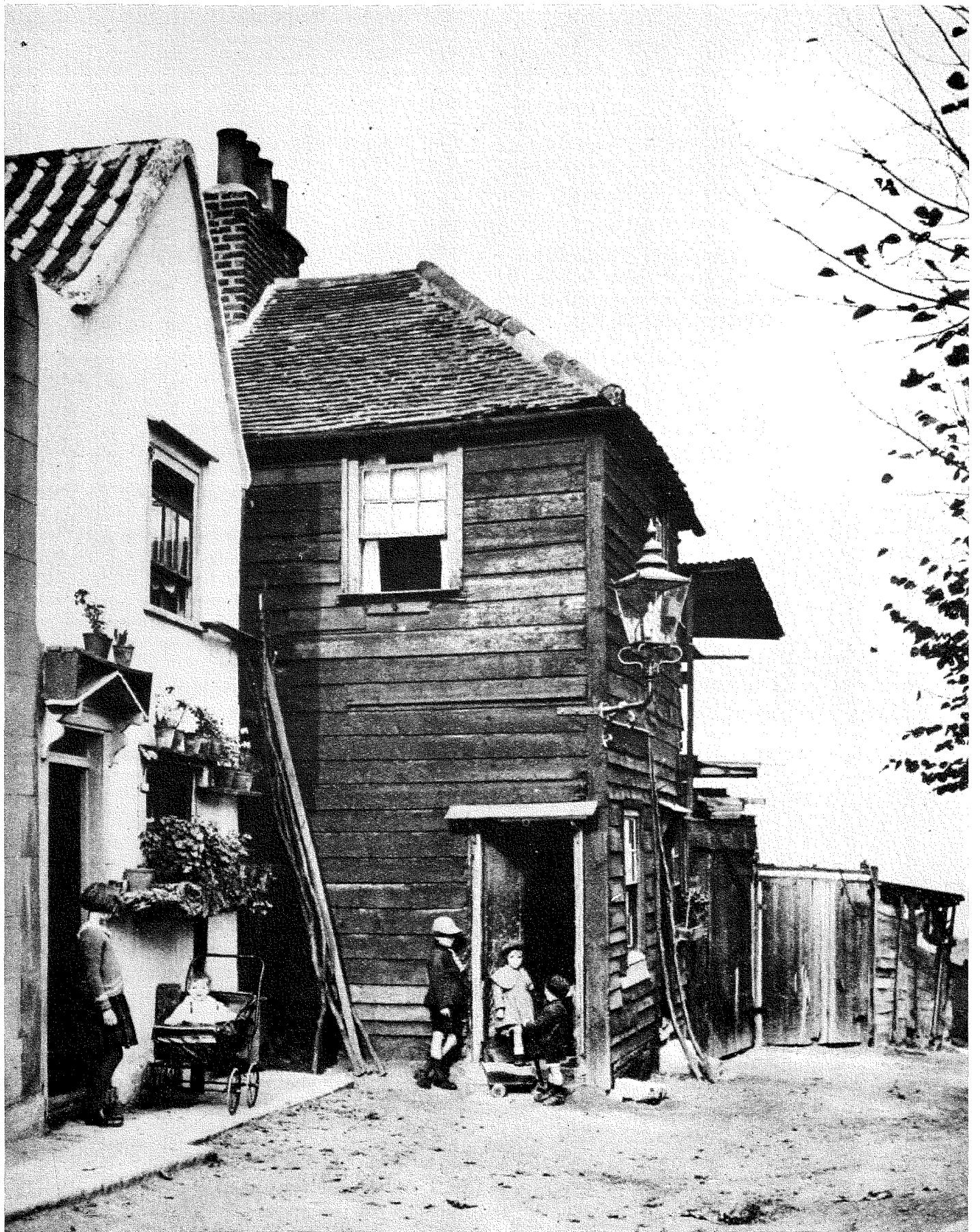
This view is outside Camden, but only just. It shows the tumble-down cottages of Townsend's Yard, on the north side of Highgate High Street - the little road that runs down to the Garden Centre, as it appeared in the 1920s
