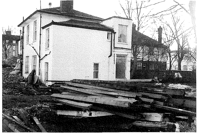
Demolition in progress at Leighton Road.
