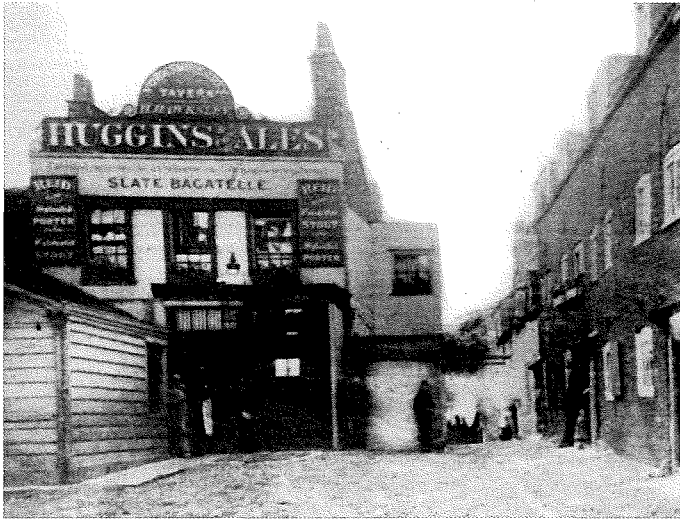
2. The Yorkshire Grey Tavern, Hampstead, photographed in 1880, a few years before its demolition for the southern extension of Heath Street. (Camden Local Studies and Archives)
