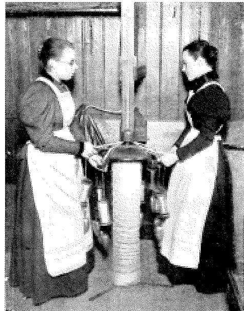
Ropemaking at the Blind School
