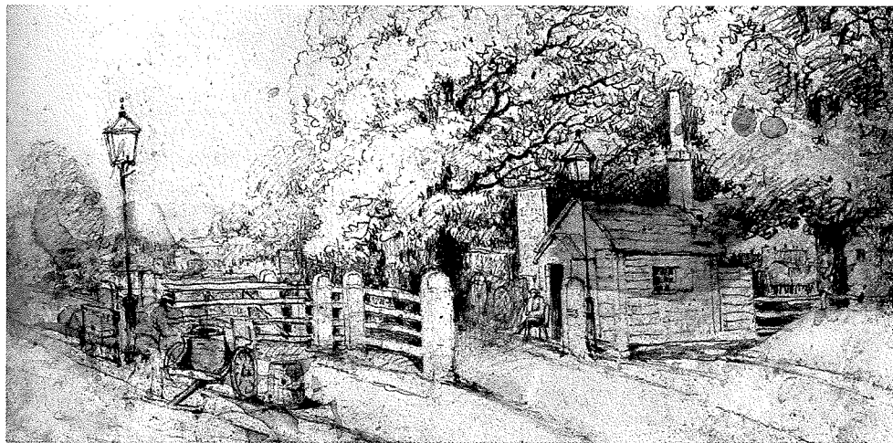
Kentish Town tollgate in 1849. It stood across Kentish Town Road near Holmes Road. The illustration comes from an undated, limited edition 2-volume work entitled Turnpikes and Toll-bars by Mark Searle
